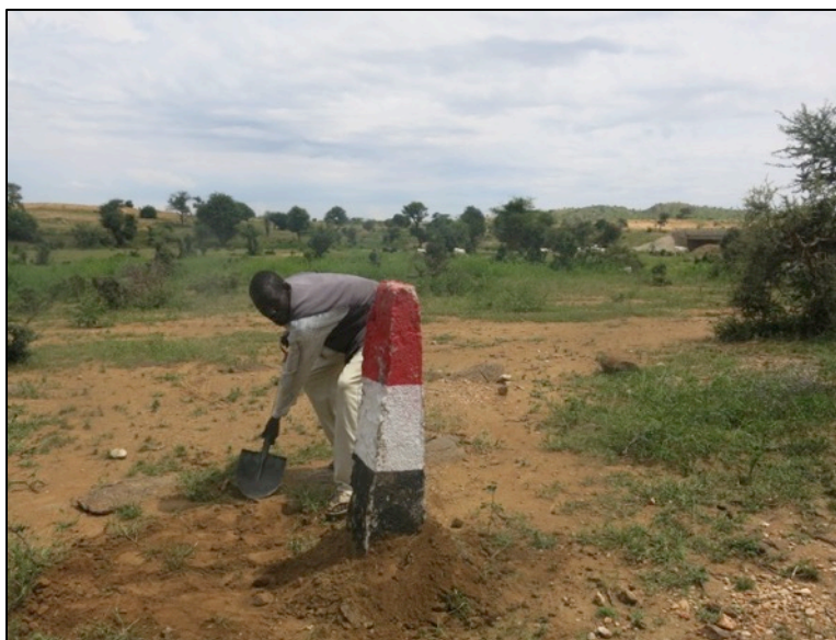
Installation of edge markers in Somei Village, near Zalingei.
