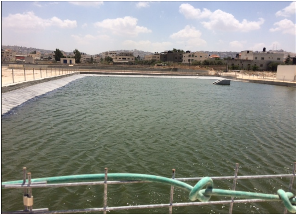
Earth pond reservoir constructed by ANERA through funding from OFID.
