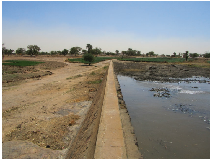
Simple dams capture rainwater runoff to support agriculture and livestock while improving infiltration and groundwater levels. (Photo: NEF)
